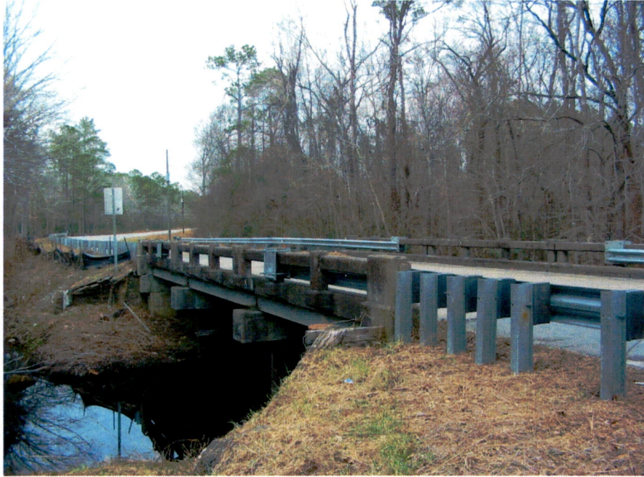
Bridge No. 104 (No. 3).
