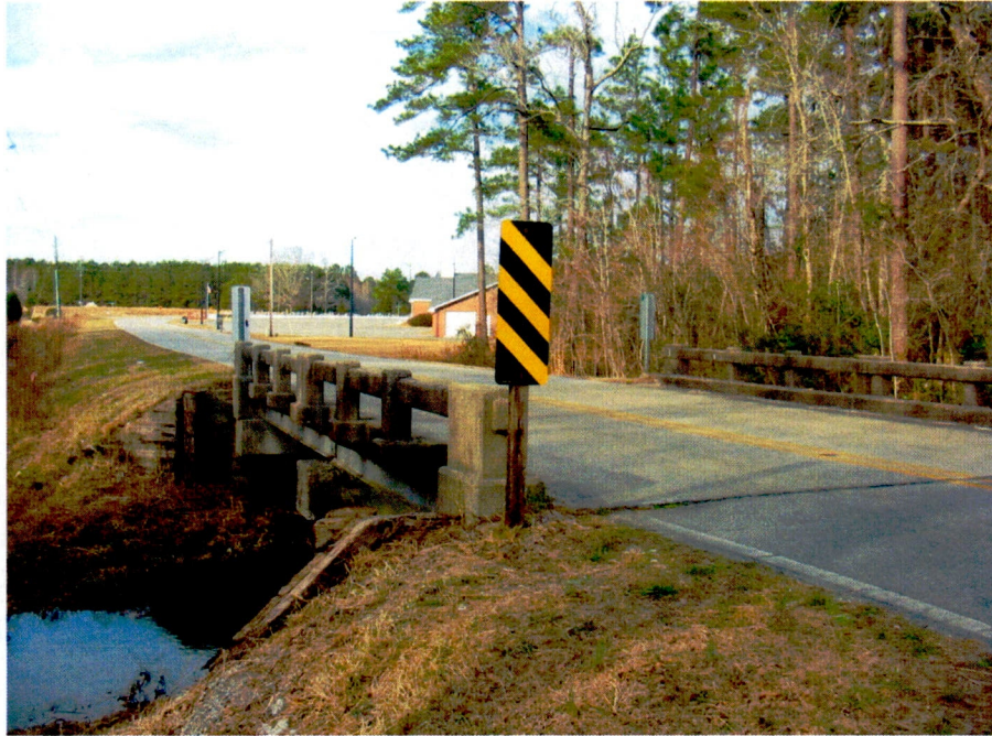
Bridge No. 23 (No. 14).
