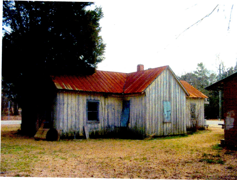
Plate 3. Antioch Crossroads Stores (Nos. 7-8), Store No. 7, (Side) North Elevation, Looking South.
