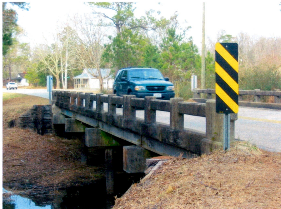
Bridge No. 25 (No. 12).
