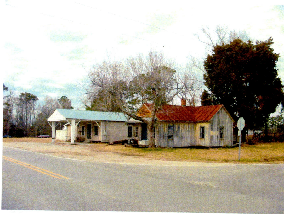
Plate 1. Antioch Crossroads Stores (Nos. 7-8), Stores and Setting, Looking North.
